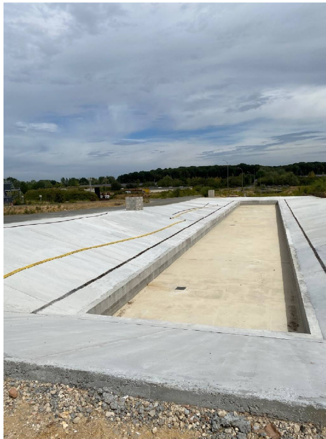
Figure 4.1 Test pit on completion of construction
