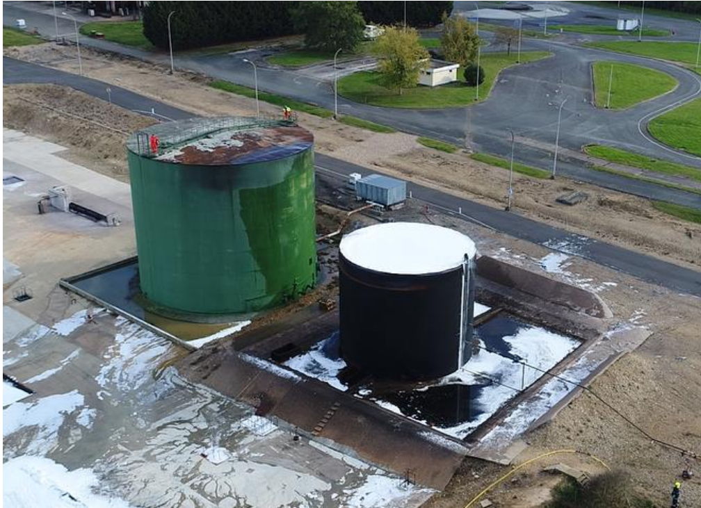
Fig. 11 Steam reduced as tank edge cools
