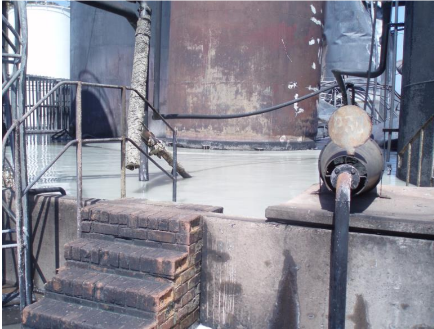
Figure 1. Example of a bund following a fire event with product and foam
