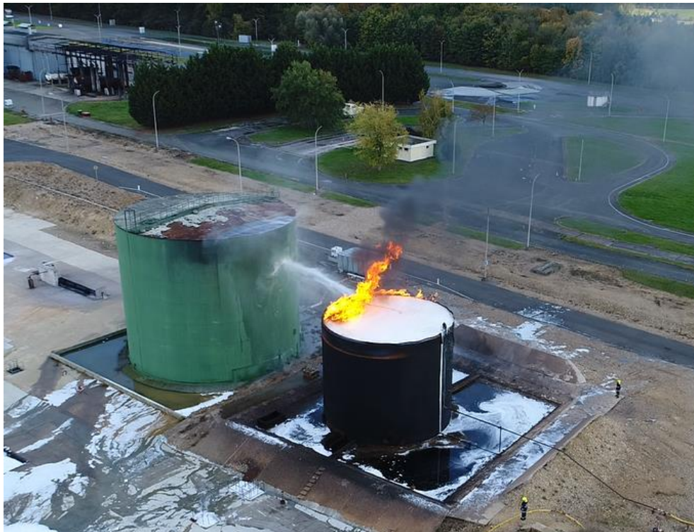
Fig. 5 Note edge sealing as foam progresses
