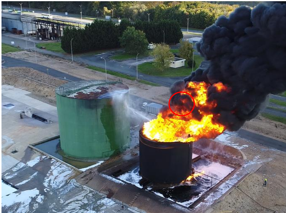
Fig. 1 Note system pourer in smoke/flame Smoke ingress can have severe effect on foam production
